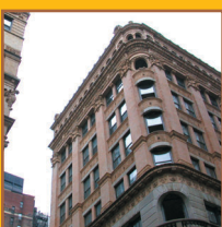
3 Fulton Building, 130 Fulton Street (Delenos & Cordes, 1891-93) The unusual rounded corner of this limestone and brick building is accented by an ornamental roofline
