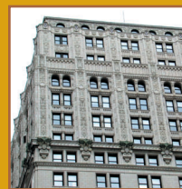
7 Electric Bond & Share Company, 2 Rector Street (Clinton & Russell, 1905-07) Ornate terra-cotta designed by architects who helped shape the character of Lower Manhattan
