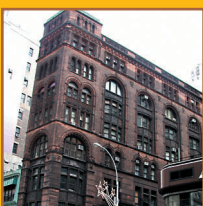
1 Corbin Building, 11 John Street (Francis H. Kimball, 1888-89) One of the area's earliest and handsomest skyscrapers with elaborate terra cotta details by Lower Manhattan's preeminent architect
