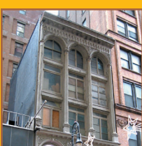
4 63 Nassau Street (attributed to James Bogardus, 1860s) An ornate facade attributed to the first manufacturer of cast-iron buildings in New York
