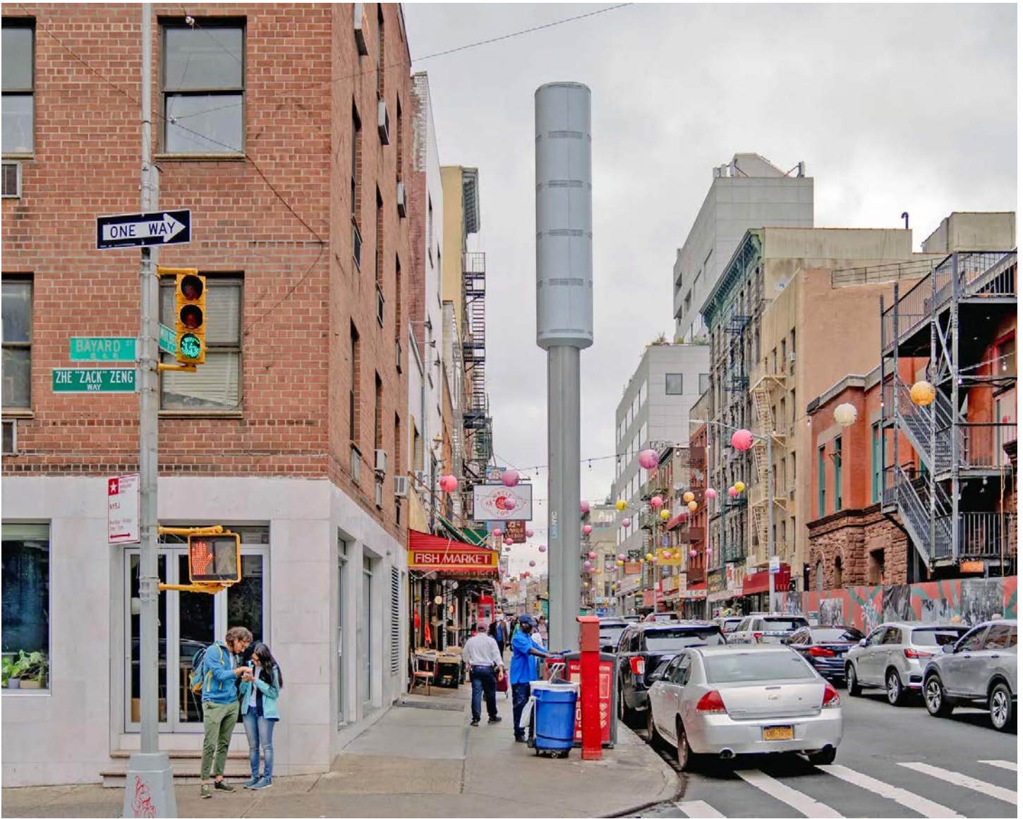
A new 5G tower on Mulberry Street in Manhattan's Chinatown (photo: Amir Hamja for The New York Times)
