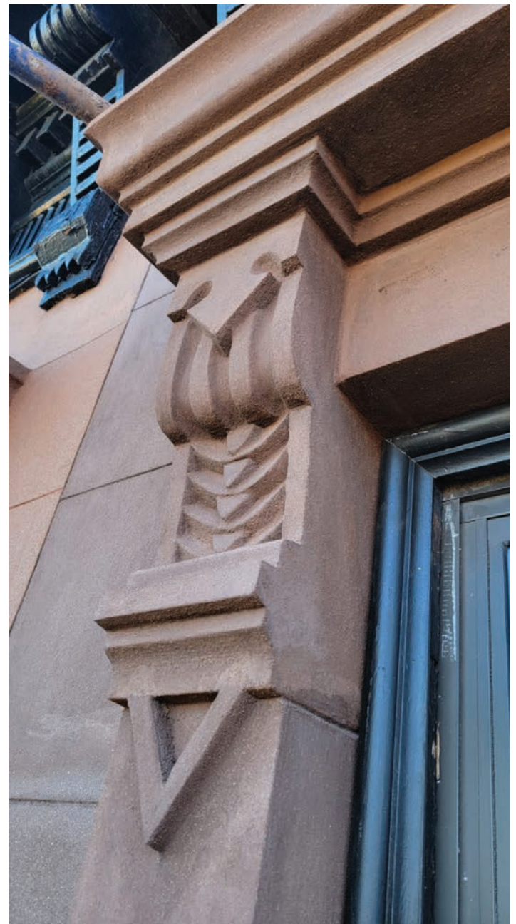
Restored brownstone at 428 Greene Avenue, Brooklyn
