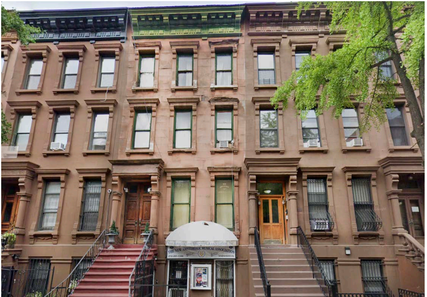
New Amsterdam Musical Association building (with awning) in 2021 before the City put up a sidewalk bridge
