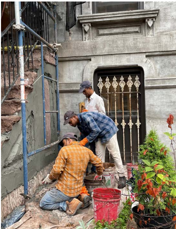
Restoration work at 428 Greene Avenue, Brooklyn
