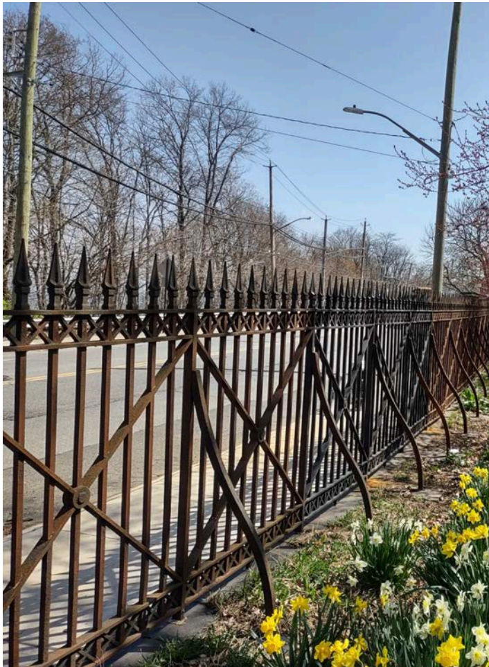
Sailors' Snug Harbor Fence Repair, Staten Island
