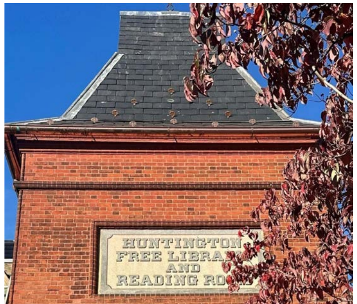
Slate Roof Restoration at Huntington Free Library, Bronx
