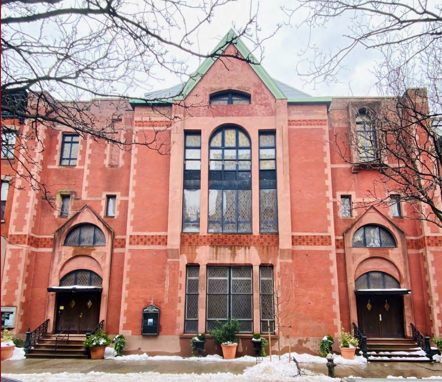
Manhattan Seventh Day Adventist Church West Village, 1882, Lawrence B. Valk, architect Foundation Repairs and Shoring
