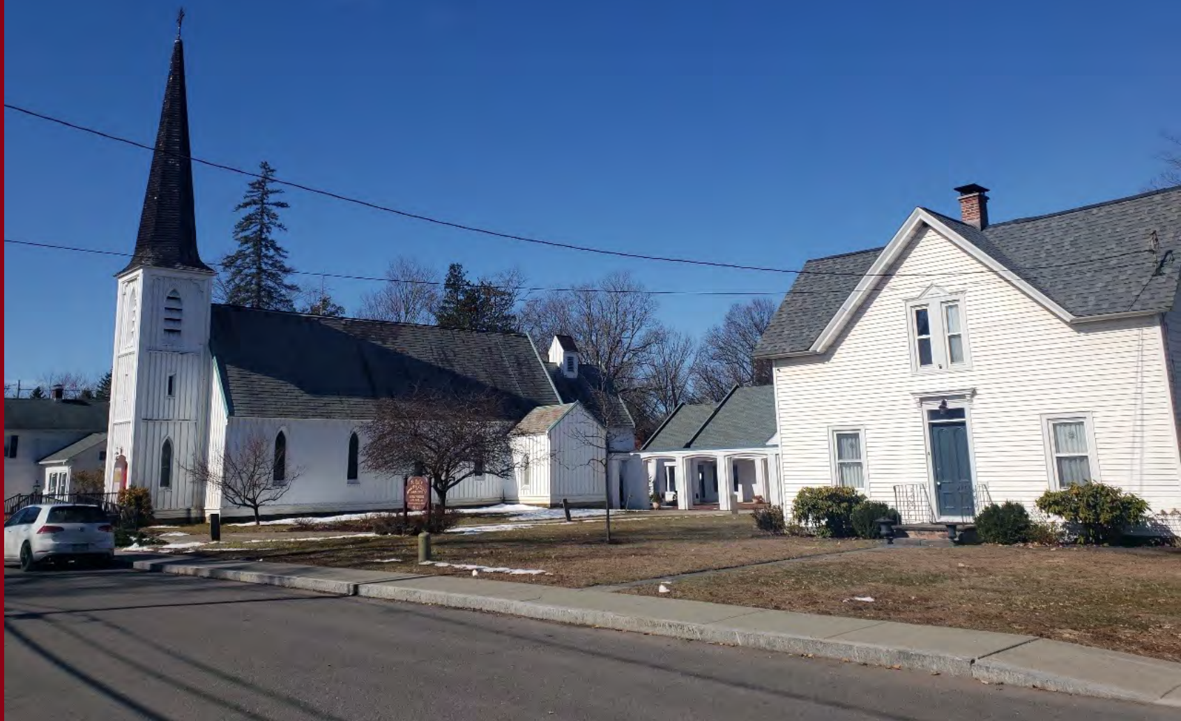
St. Paul's Episcopal Church Kinderhook, 1851, Richard Upjohn Sacristy Roof Replacement, Basement Bulkhead Reconstruction
