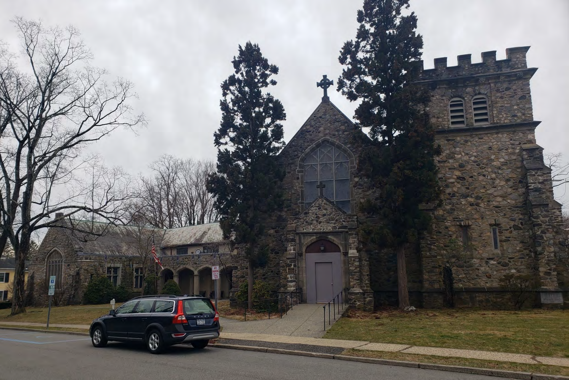
St. John's Episcopal Church Pleasantville, 1912-1914, Charles A. Hoag, architect Steel Window Restoration
