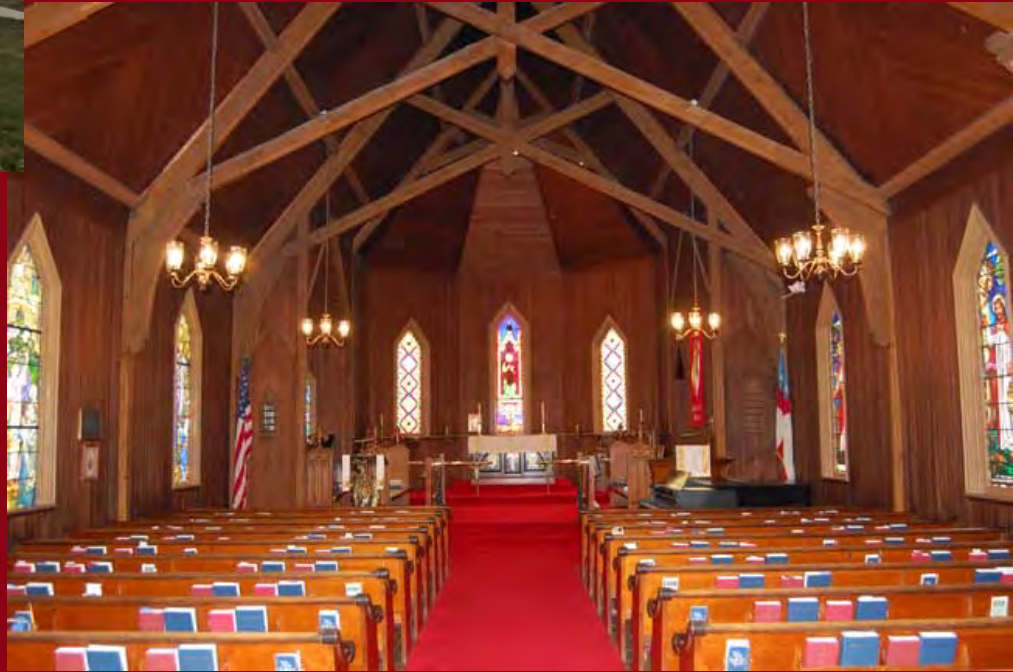
St. John's Episcopal Church Youngstown, 1878, Richard M. Upjohn (attributed), architect Roof and Gutter Repairs, Foundation Repointing
