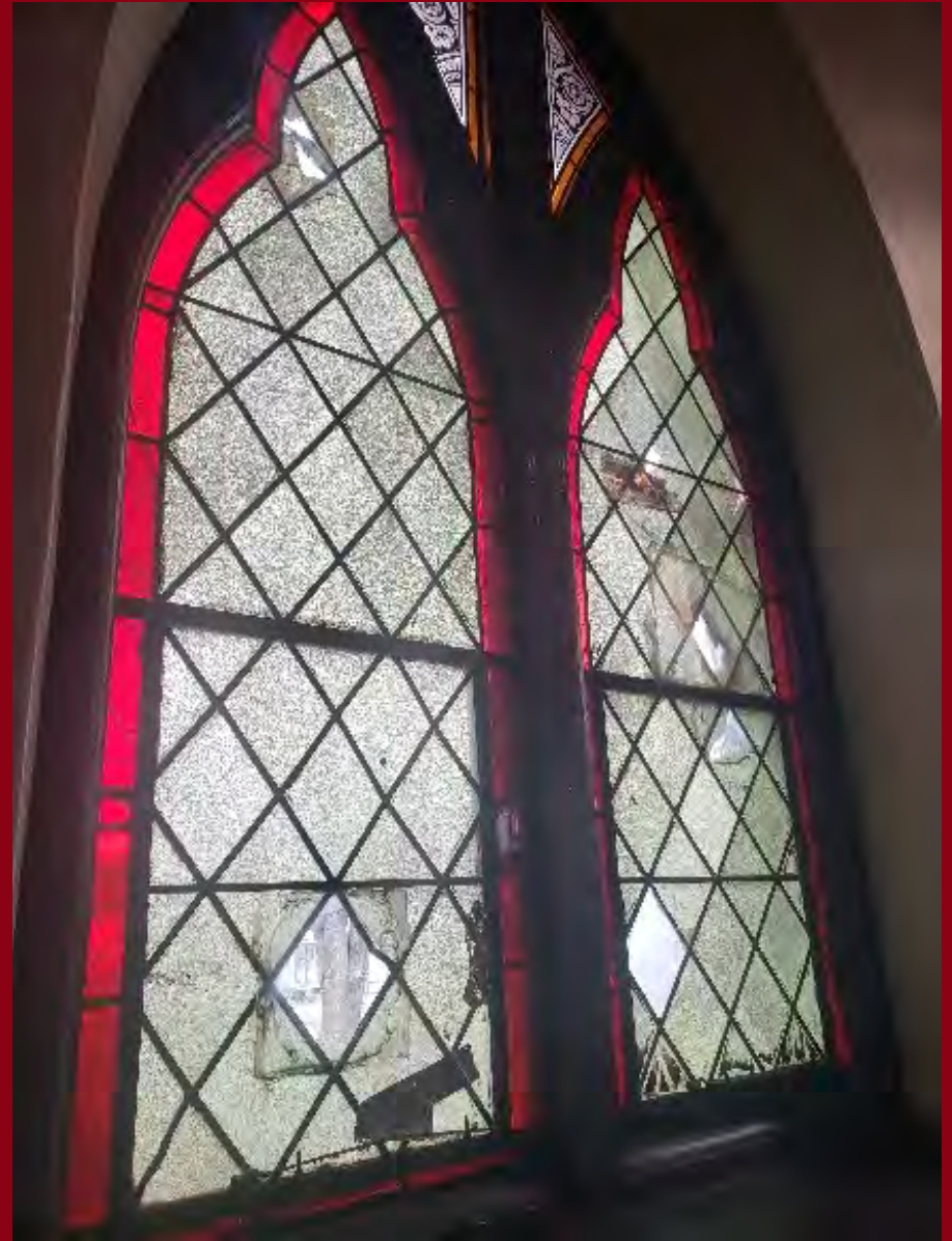
St. Paul's Episcopal Church Conditions Survey
