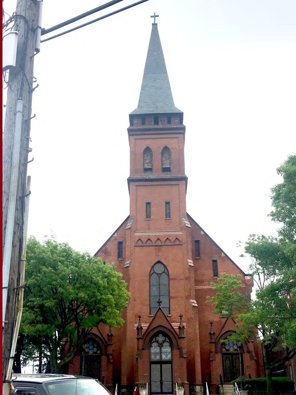
St. Raphael Roman Catholic Church Long Island City, 1881, attr. Patrick Keely, architect Roof Replacement
