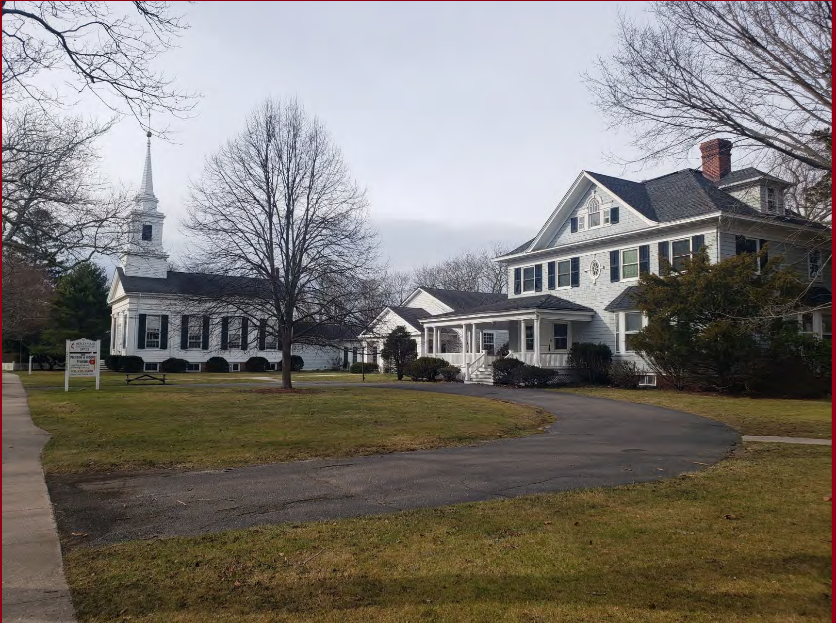
Bellport United Methodist Church Bellport, 1850, Hulse Brothers and Charles Hallock, architects Conditions Survey
