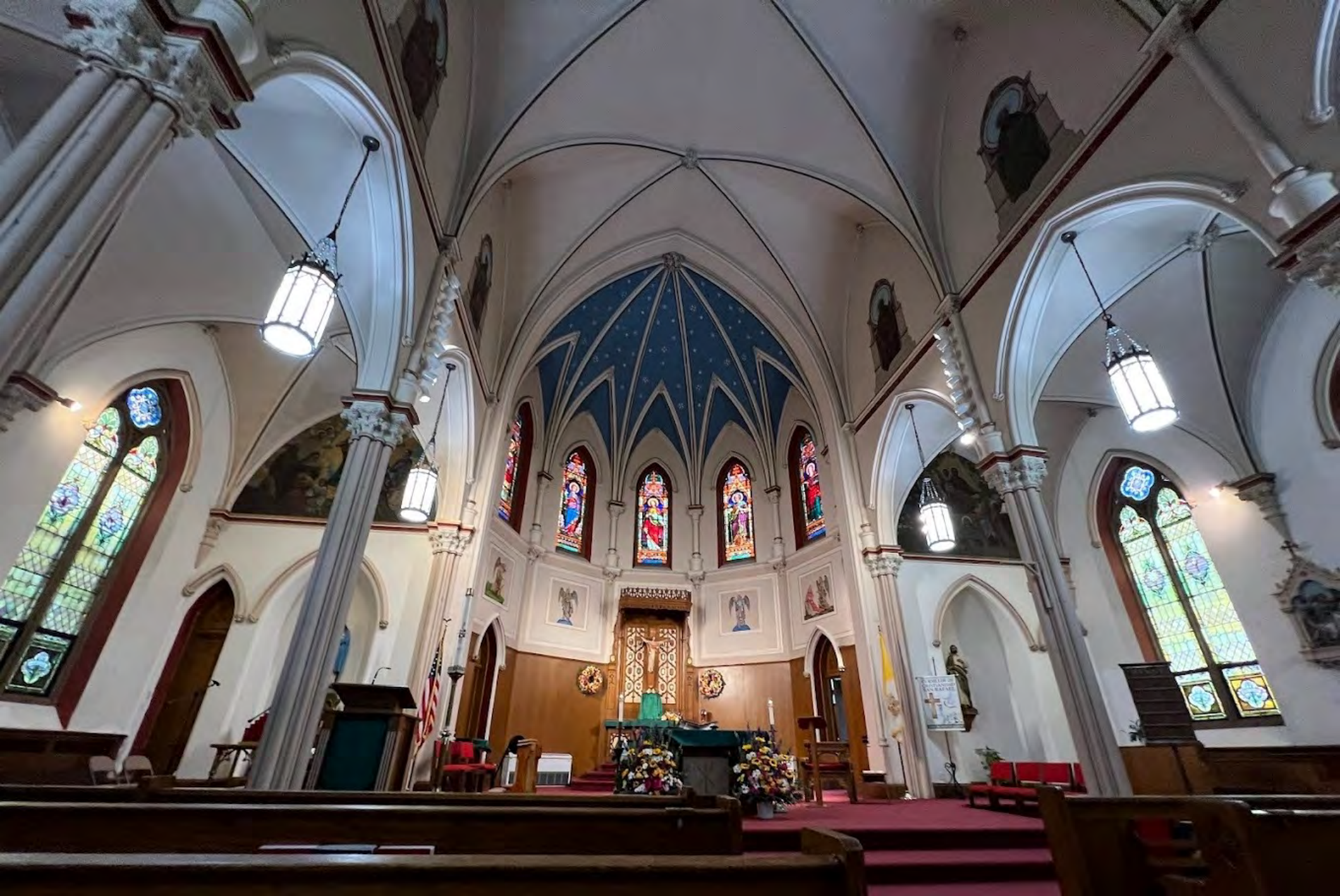
St. Raphael Roman Catholic Church Roof Replacement
