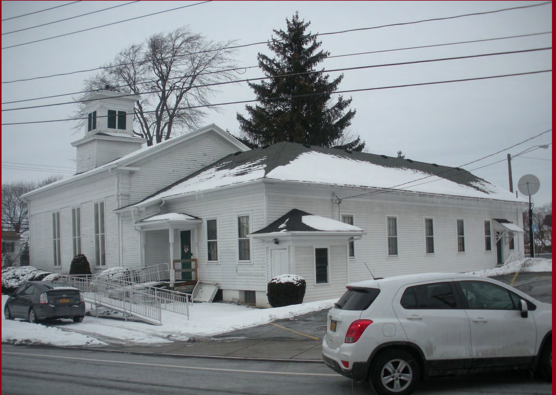
West Henrietta Baptist Church Fellowship Hall Roof Replacement
