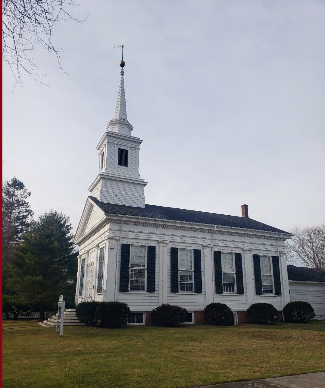
Bellport United Methodist Church Bellport, 1850, Hulse Brothers and Charles Hallock, architects Conditions Survey
