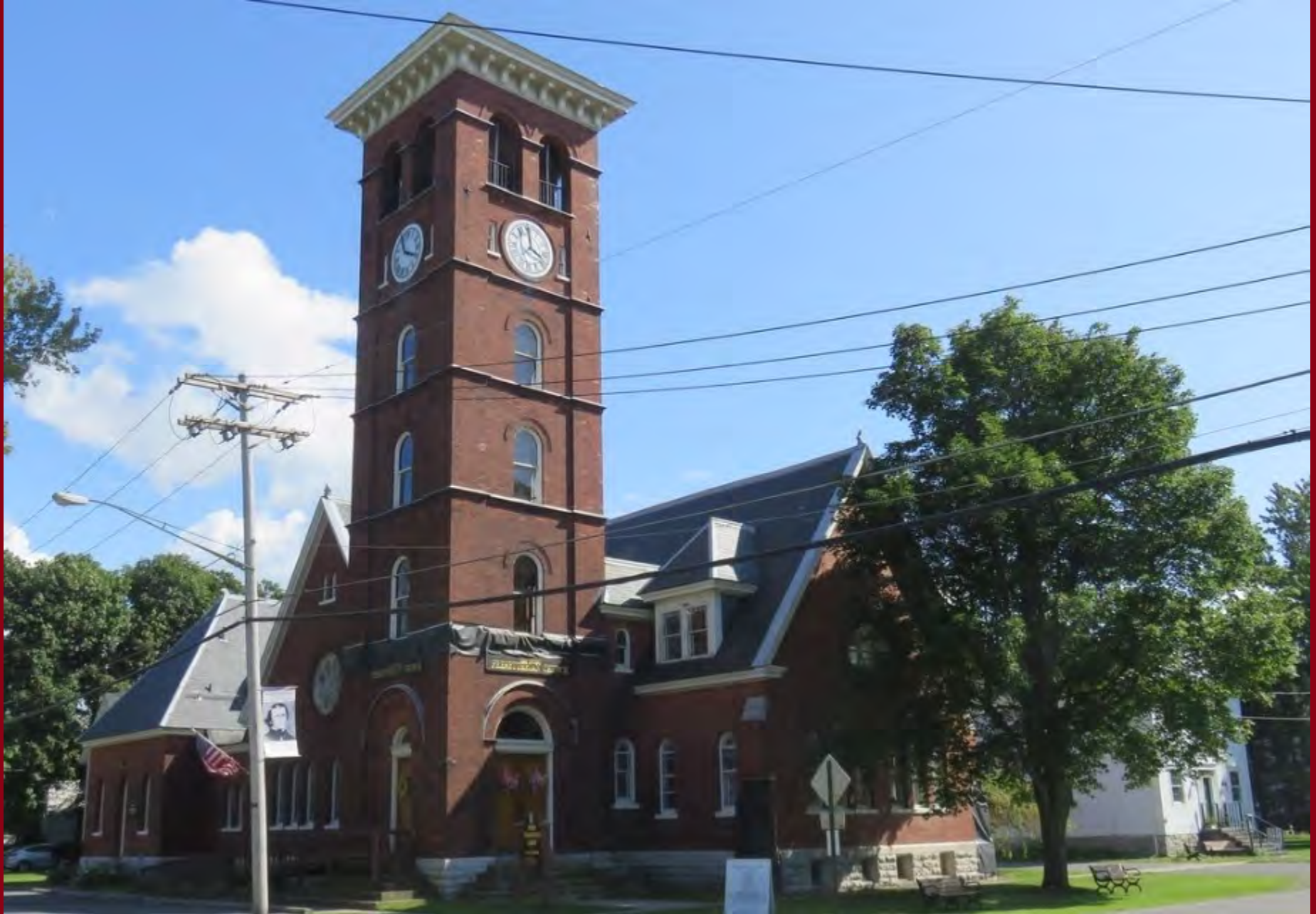
United Presbyterian Church of Sackets Harbor Sackets Harbor, 1900, D.D. Kieff, architect Tower Repairs
