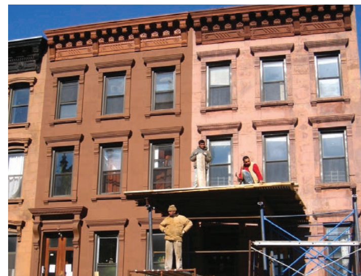
Repair work at 329 and 331 MacDonough Street
