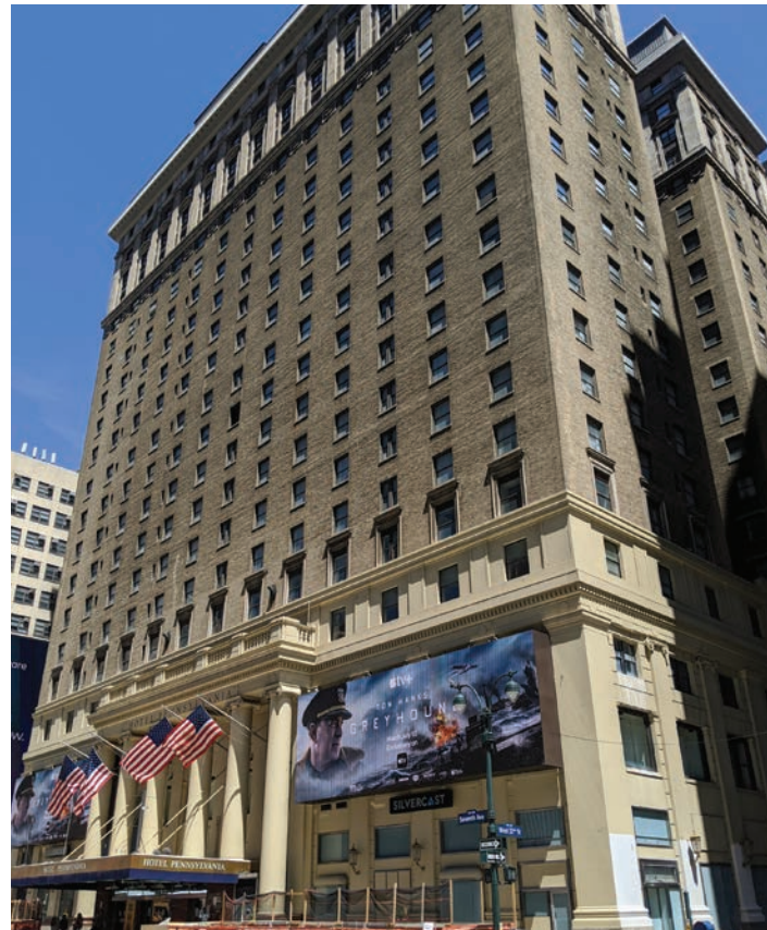
Opened in 1919, Hotel Pennsylvania at 401 Seventh Avenue was once the largest hotel in the world. It closed in 2020 and is being demolished to make way for Penn15 Tower
