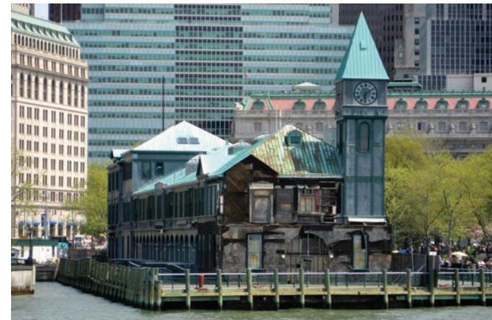
Pier A, Battery Park, Lower Manhattan, before restoration, 2008
