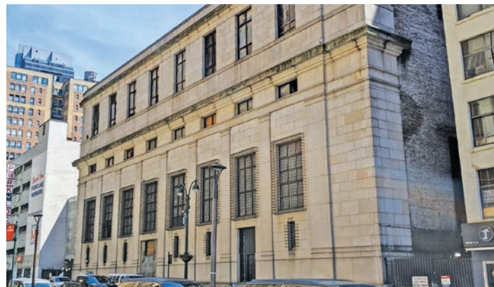
Penn Station Service Building, 236-248 West 31st Street
