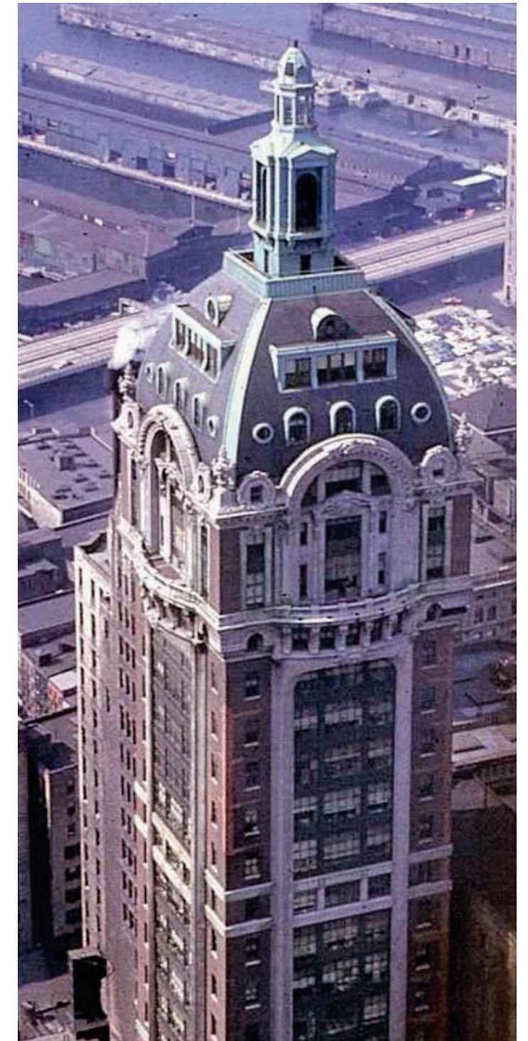
Ernest Flagg's splendid Singer Tower, 1906-1908, demolished 1968
