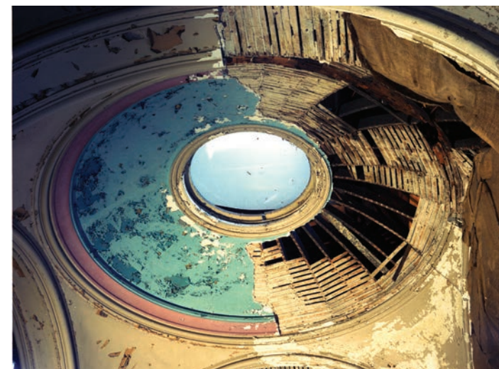
Eldridge Street Synagogue interior, before restoration
