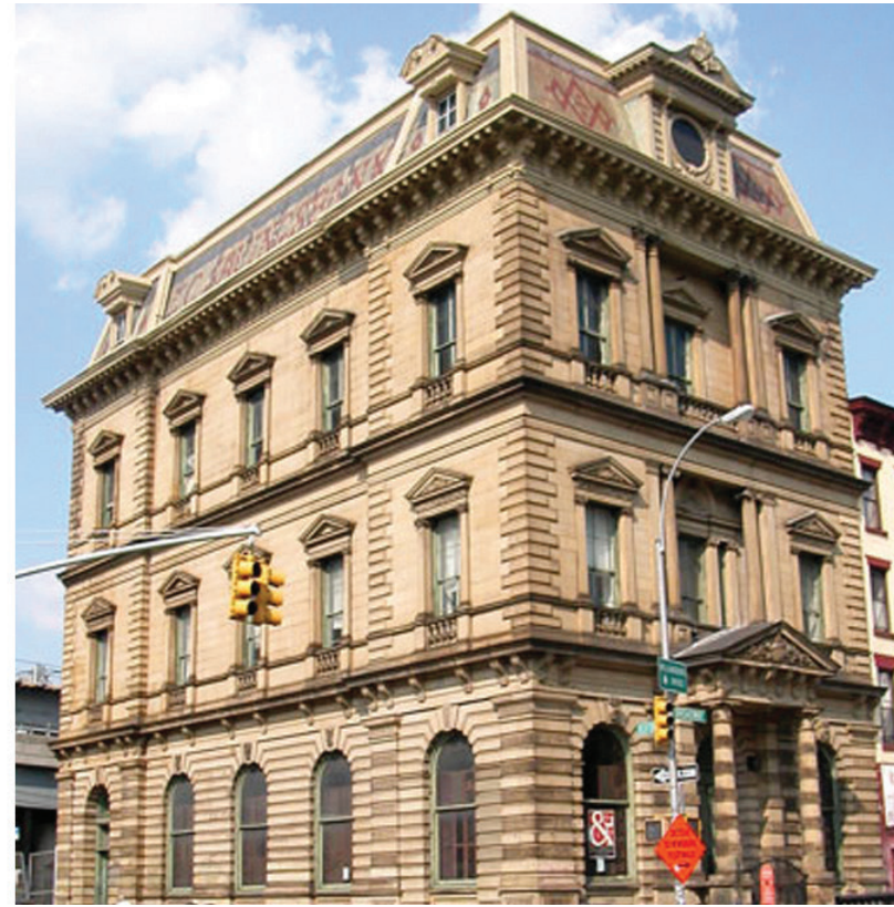
Williamsburg Art and Historical Society, clock tower dormer, before and after restoration
