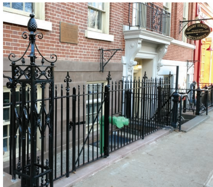
Restored railing, Henry Street Settlement
