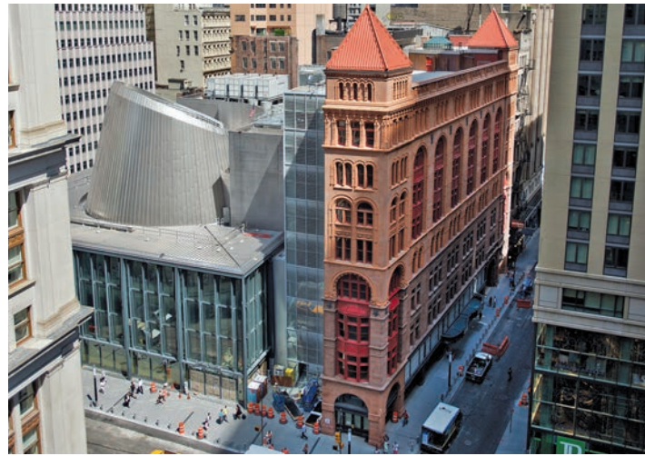
Corbin Building, 11 John Street
