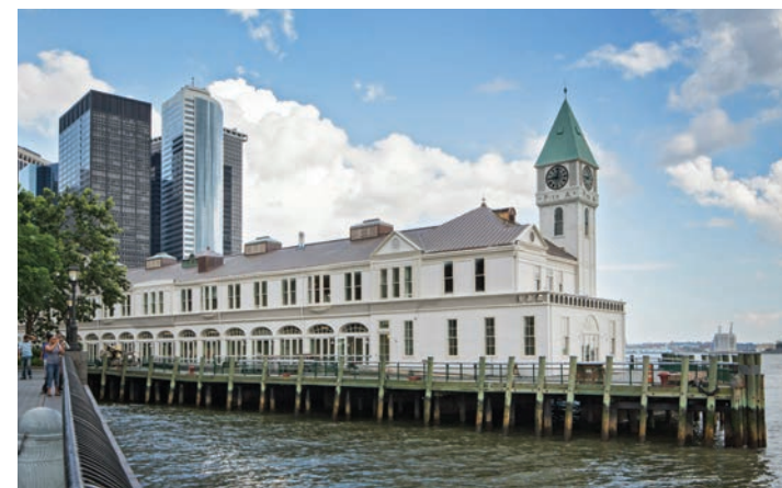
Pier A, after restoration, 2014 (photo: Hardy Collaboration Architecture)
