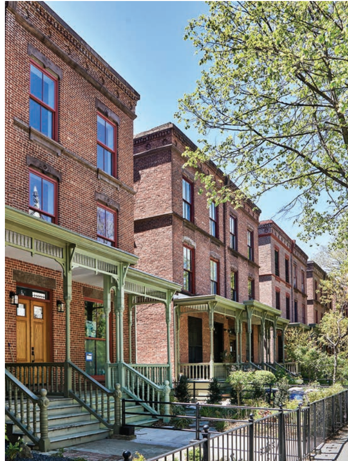
Astor Row, after restoration (photo: Noël Sutherland)
