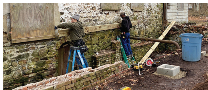
Olmsted House, work in progress
