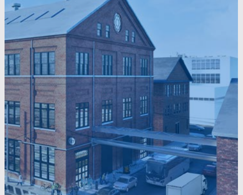
31st Annual Preservation Award Winner - Brooklyn Navy Yard Building 127 Rehabilitation
