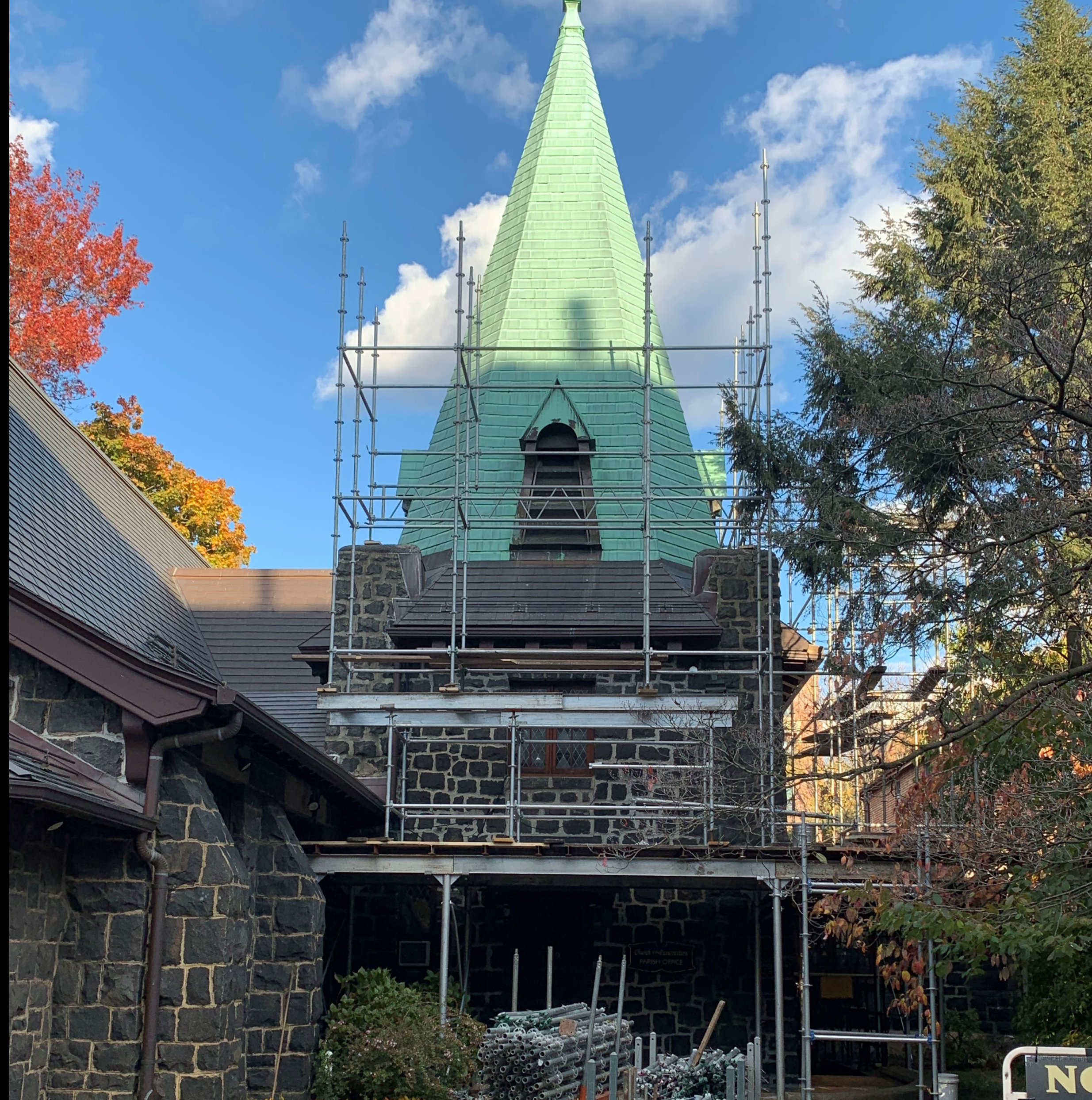
Church of The Resurrection, 1874, 1905, Kew Gardens, Queens Henry Dudley (1813-1894), Nathaniel W. Vickers (1846-1947), architects Copper Tower Roof Restoration
