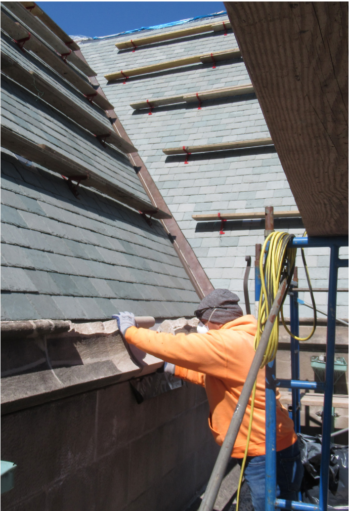
Coping stone reinstallation, Fourth Universalist Society, Central Park West.
