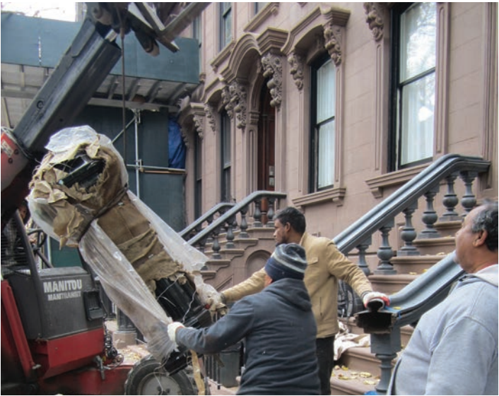
Installation of one of the new newel posts at 6 South Portland.
