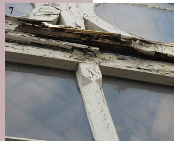
7 Historic window condition prior to restoration, detail of weather rotted mullion
