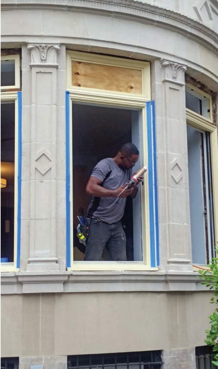
Contractor installing the windows at 299 Lefferts Avenue
