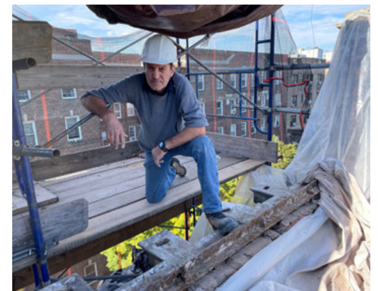
Inspecting parapet after removal of terra cotta
