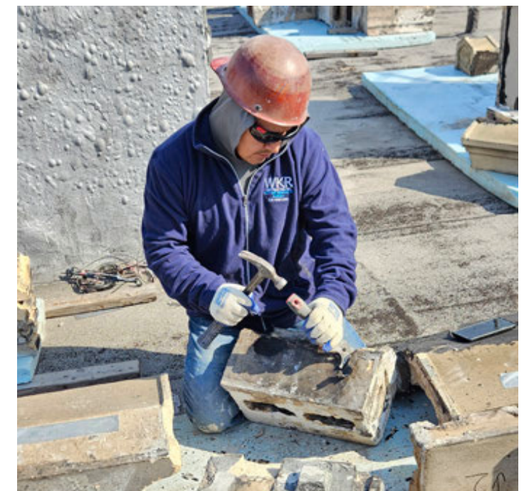
Cleaning original terra cotta for reuse
