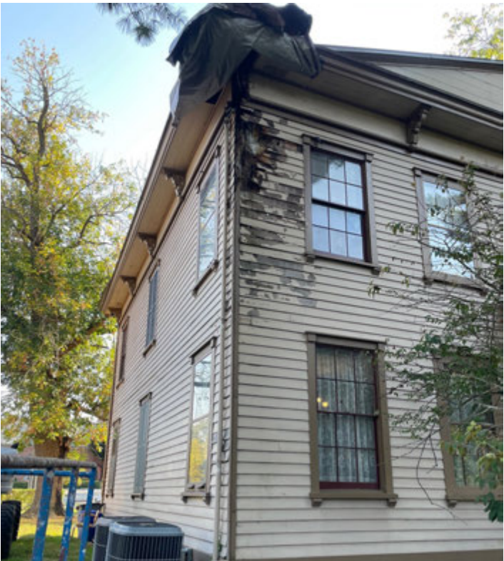
Stephens-Prier House wood deterioration
