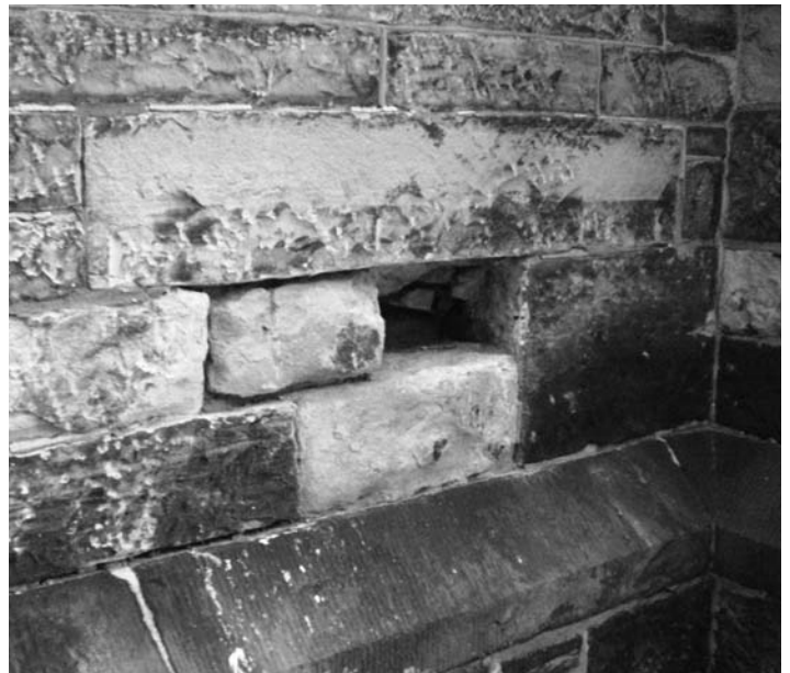
Above and below: The 1853 Richard Upjohn-designed Christ Episcopal Church in Binghamton has had masonry problems for years; missing and delaminating stones characterized its façade. Opposite page: The United Church of Cohoes was built in 1865.
